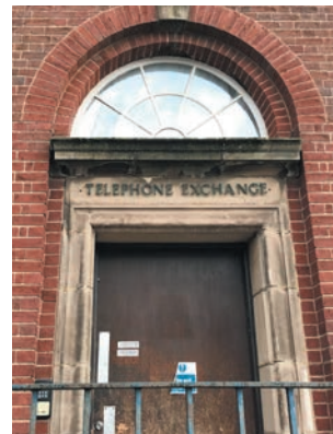
The Priory Telephone Exchange
