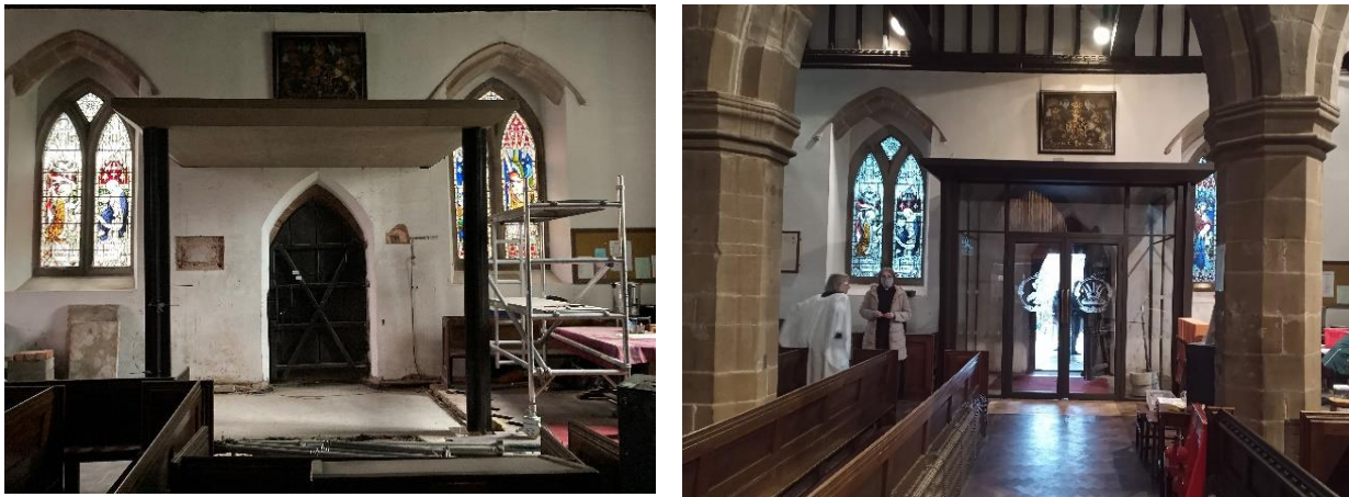
Figure 8 - Porch frame and after completion with glass panels
