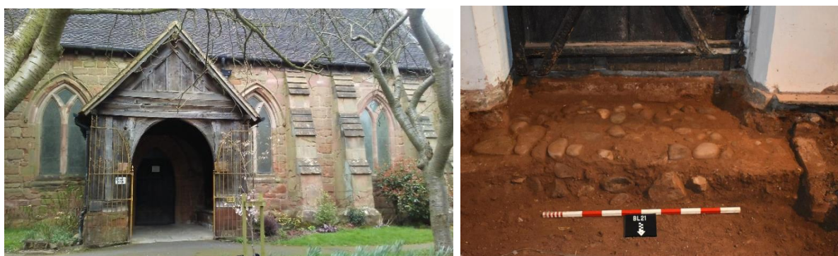
Figure 7 – External porch and cobbled footing inside the doorway (Photo - Archaeology Warwickshire Report2110).
