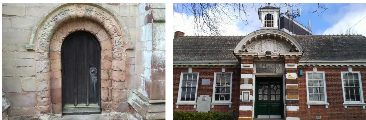
Figure 4 - Norman door St Laurence Church & Northfield Library
