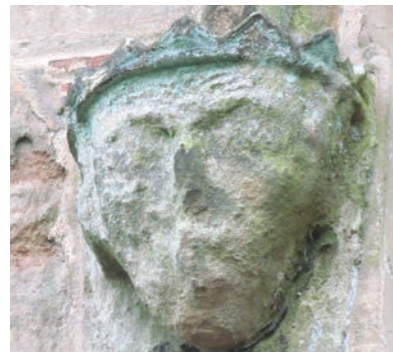
South Aisle east window, much eroded. There are better preserved figures in the outer porch and on the tower arch.
