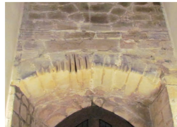
Grooves worn by the rope from a bell once hung above the door.
