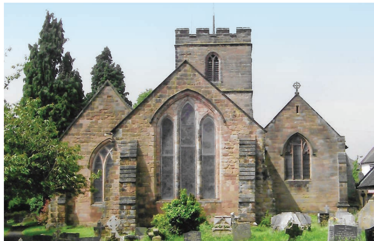
A view from the east, with the huge lancet windows and clapping buttresses of the chancel, the south and north aisles and the tower. The dripstones above the chancel and south aisle windows have much eroded carved heads at their ends, possibly of kings and queens.
