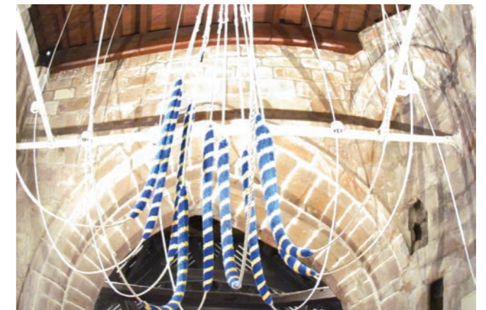
The bell ropes are dropped through the roof and held in a safe position in the frame. They are lowered by a rope and pulley "spider" when they are to be rung.
