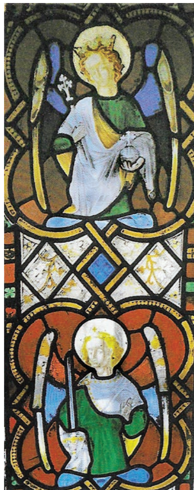
Pugin Window undergoing restoration at Hardman's Studios, 1995.
