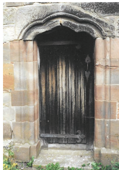
Priest's door to the chancel. Now blocked on the inside.
