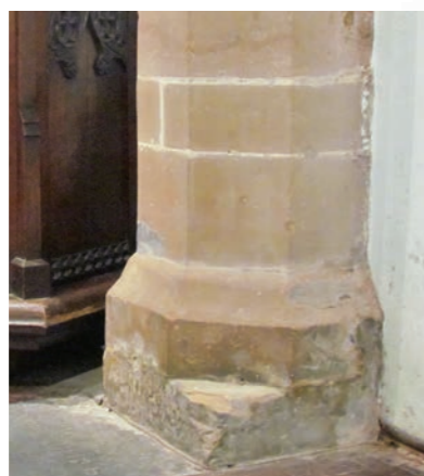
East end column exposed stonework.
